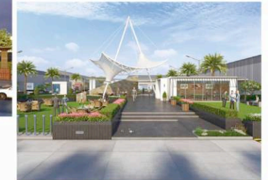
Indraprasth Industrial & Logistics Hub (Warehouse)
